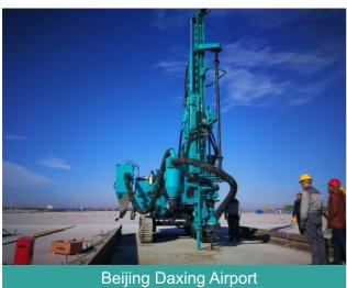
Special drilling equipment SWDE120R by adopting geothermal conduction technology, the futuristic technology of helping geothermal melting snow.
